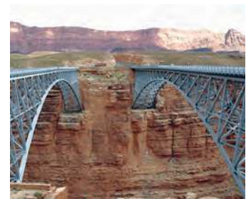
Hoover Dam Bridge
